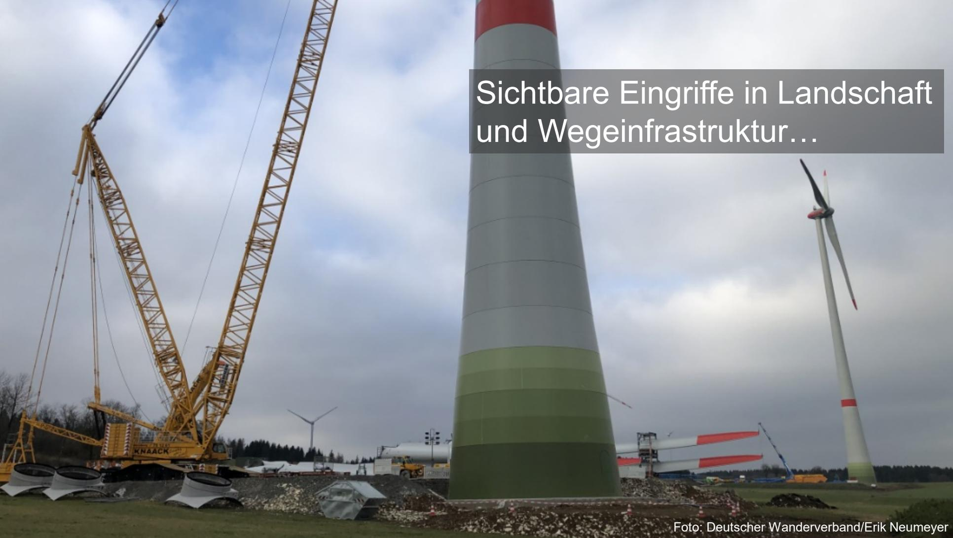
A large-scale construction site for a wind farm. In the foreground, a tall, grey concrete tower is being built, featuring a red band at the top and a green band near the base. Two large yellow cranes are positioned to the left, with their jibs extending towards the tower. The ground is a mix of dirt and grass, with several concrete segments lying nearby. In the background, other wind turbines are visible under construction, and a cloudy sky is overhead.
